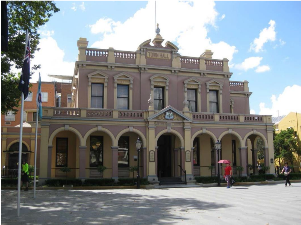
Figure 11 Parramatta Town Hall
