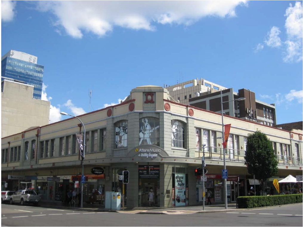
Figure 2 View of the site (corner of Macquarie and Church Streets)
