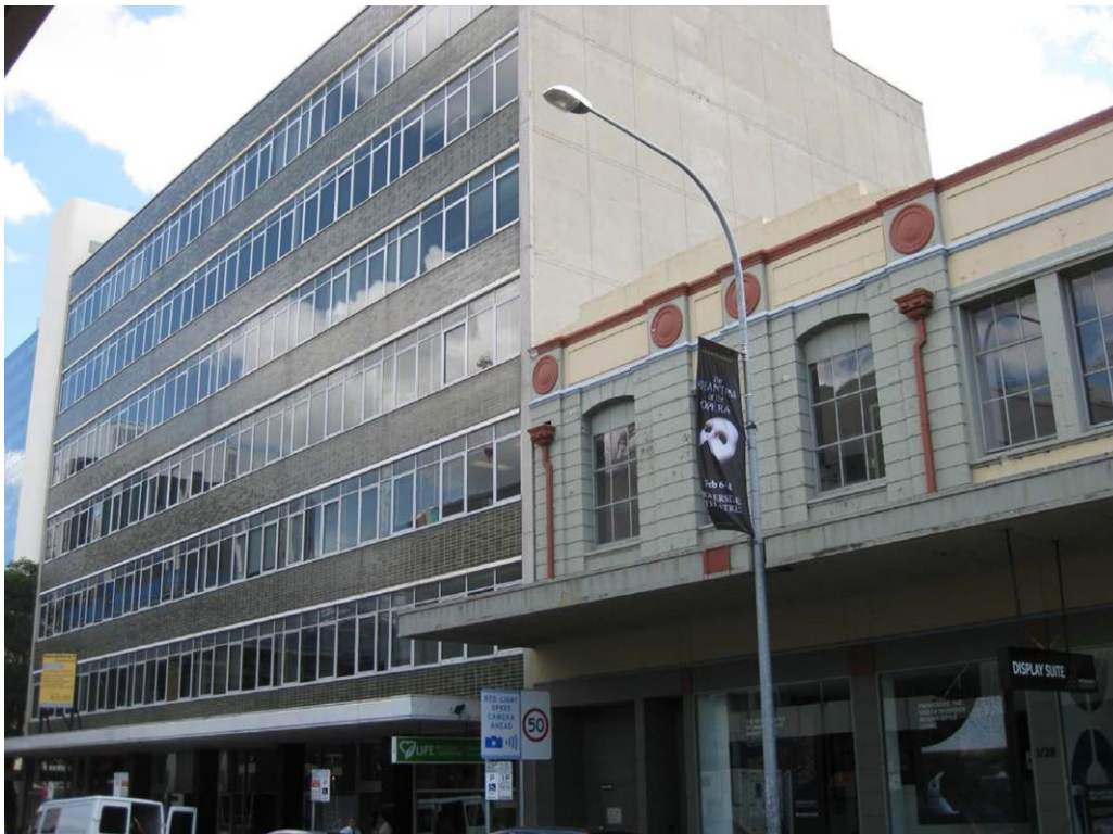
Figure 16 View of 20 Macquarie Street (adjoining the site)
