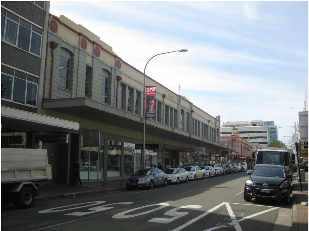
Figure 5 View of Macquarie Street frontage
